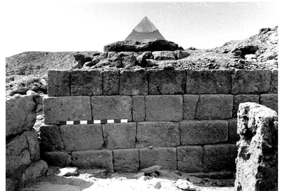
25d. 2088: stepped northern facade and the abutment of serdab 1. A roof block of serdab 1 is centered under the tip of the pyramid of Khafre; under its right end begins the stepped joint that represents the original stepped facade of the mastaba against which serdab 1 was built. At left is the southwest corner of 2086, and at right the badly weathered door of 2099. The intact serdab of 2099 was found in this corner (rg 7-28, 1989)
