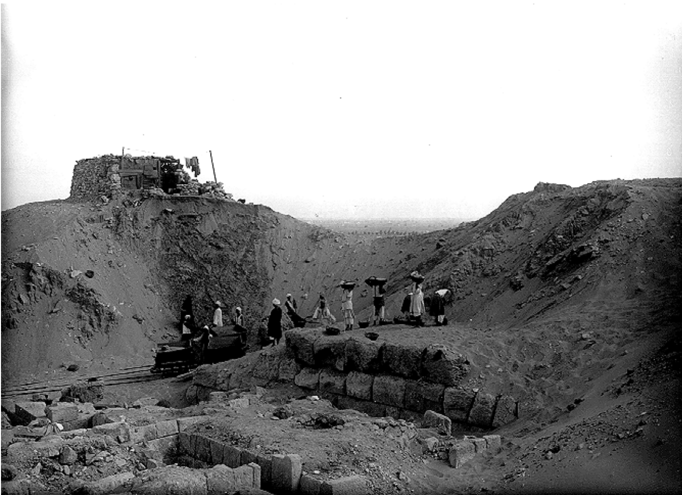
5b. The removal of the "big dump" over 2230, February 11, 1939. The jambs and corridor of 2087 are visible in the foreground. Note larger blocks ("w-masonry" of the west facade of 2230 and the extensive weathering of its top course (a 8099)
