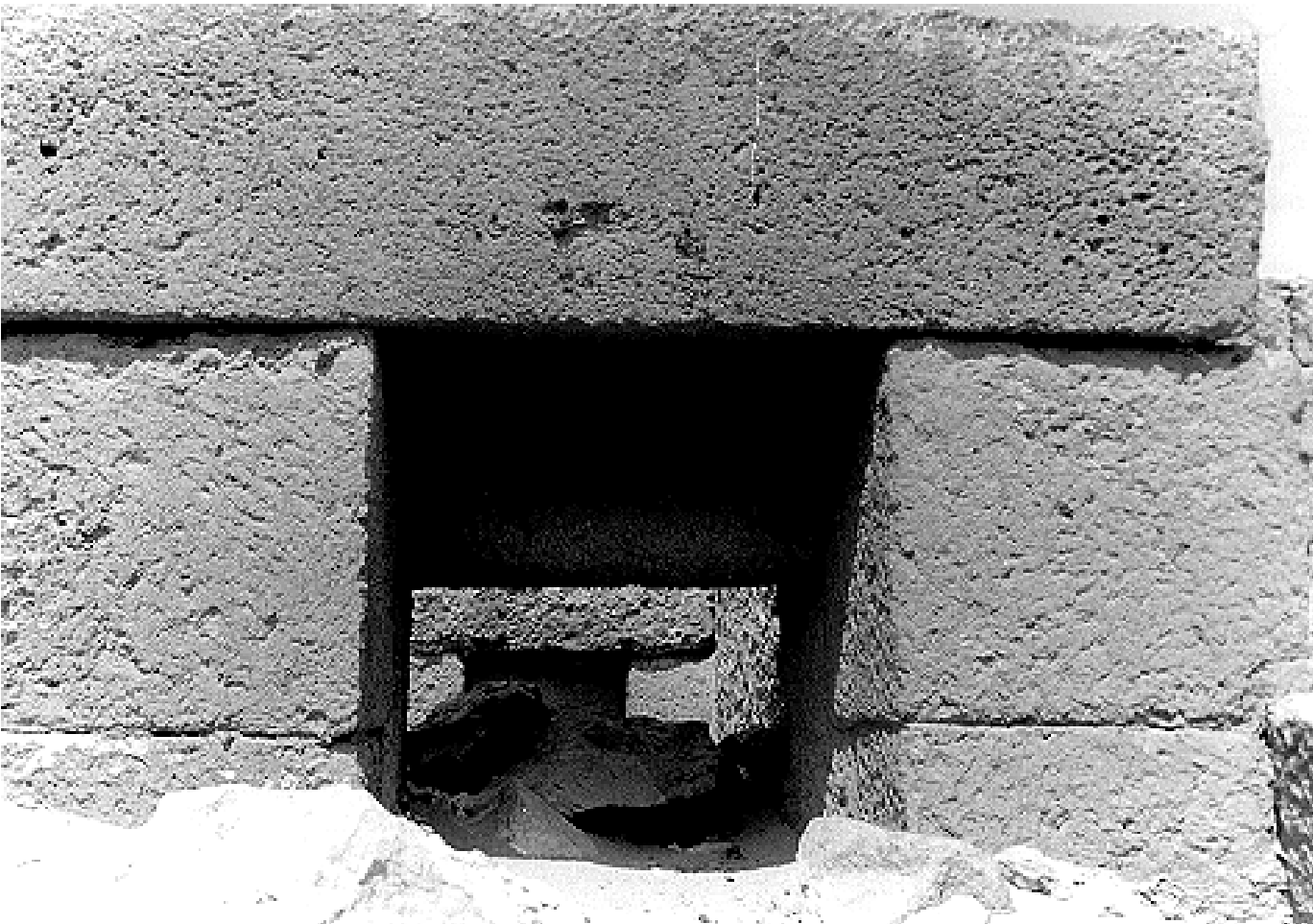
36b. 2089: view through the largely buried entrance doorway. Beneath the drum lintel, the lintel, jambs and part of the tablet of the northern false door are visible. A small opening at the top of the tablet is the serdab slot. The entrance and chapel of this tomb were buried by four intrusive shafts and burial chambers (amr, 1990)
