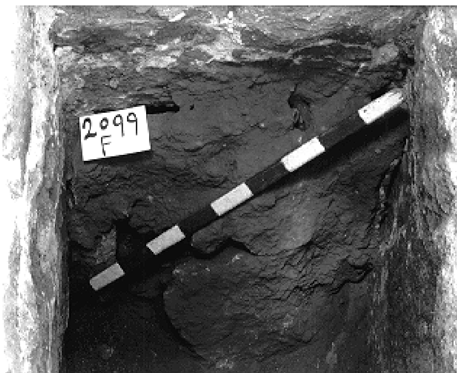
117c. 2099 f: intact blocking type vi d(2), wedge-shaped wall of rubble bound with mud (c 14264)
