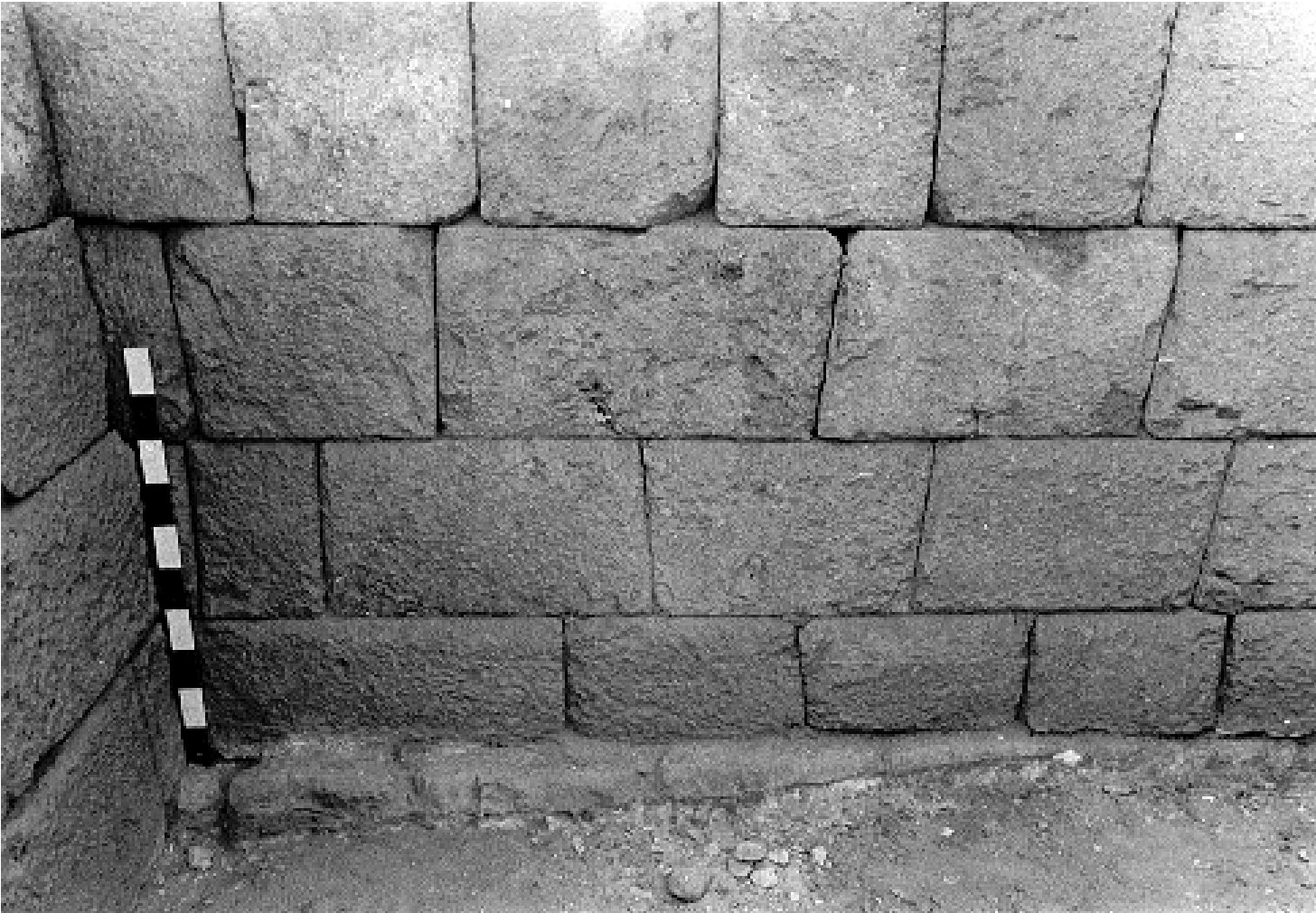
86a. 2097: corner of the courtyard to the east. The angled line at the base of the later east wall of the courtyard shows the line of the original west facade of 2097', rebuilt to make the courtyard rectangular. The wall at left is the north wall of the courtyard, added in Phase iii (rg 6-23, 1989)
