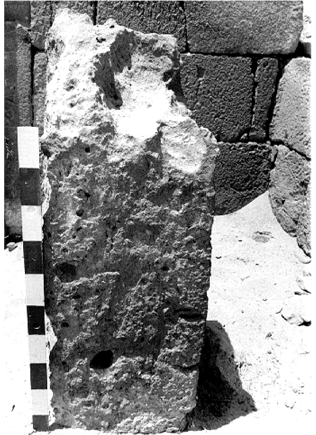
121c. 2240: north pillar of portico, east face. A standing figure in sunk relief, wearing a triangular kilt, facing left, originally decorated this pillar (rg 9-14, 1989)
