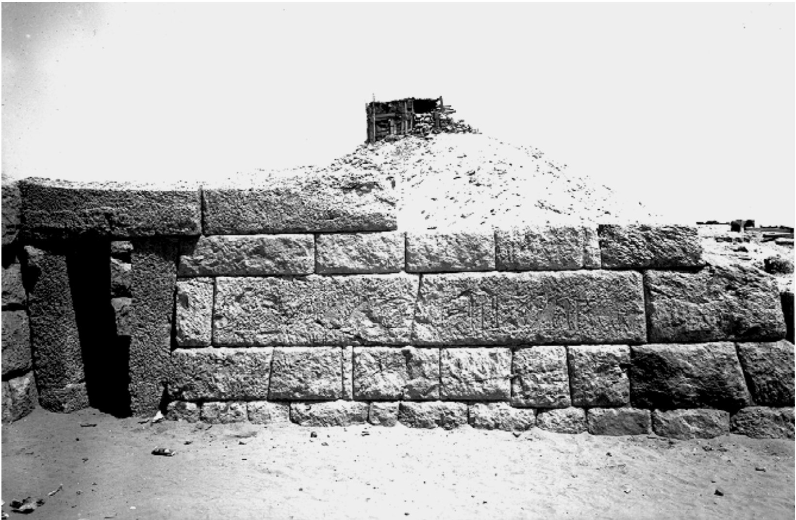
118c. 2230+2231: southern doorway and south face of 2231, with an intrusive inscription of Khuwi-Re centered on the two large blocks of the third course. The angled doorjambs and the unevenness of their join with the adjacent facades is a result of its transplantation from the northern end of the corridor in Phase iii. May 1, 1939 (a 8221, and e 3625)
