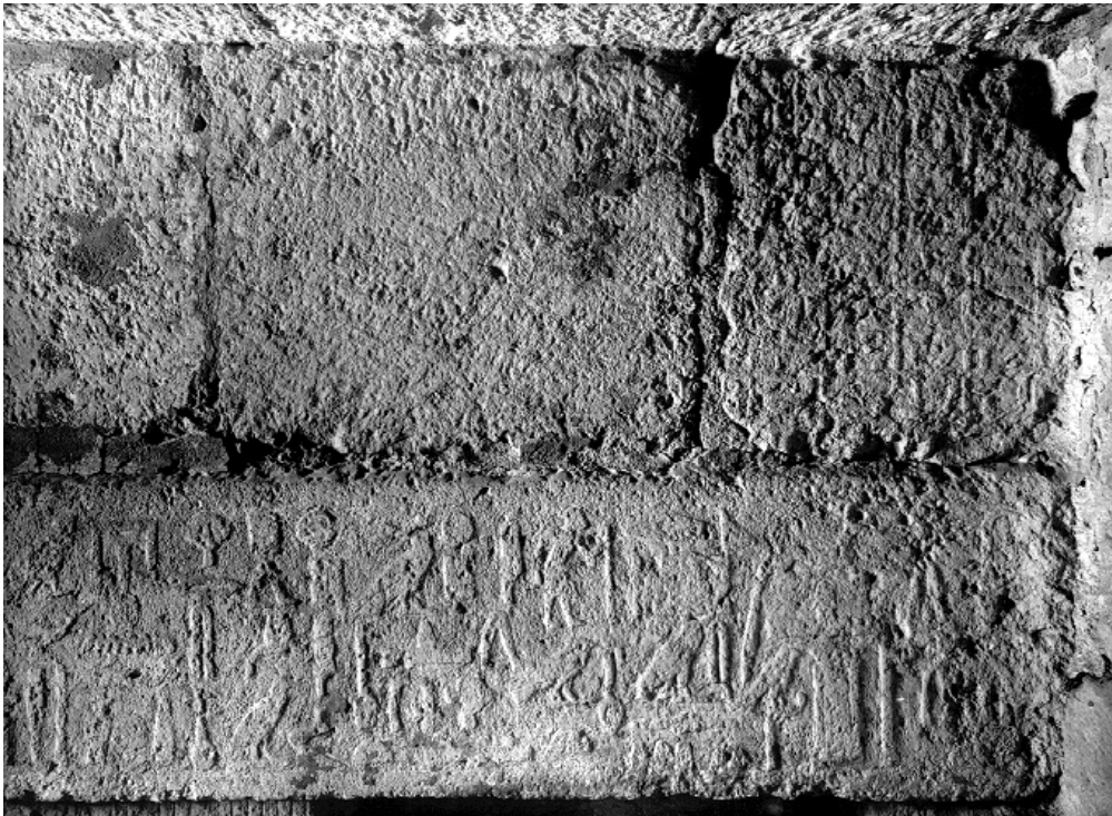
55a. 2091: north end of upper lintel surmounting the false doors, and the wall above it. Above the lintel and slightly set back from it, an offering list was planned, of which only the rightmost part was carved (a 6447)
