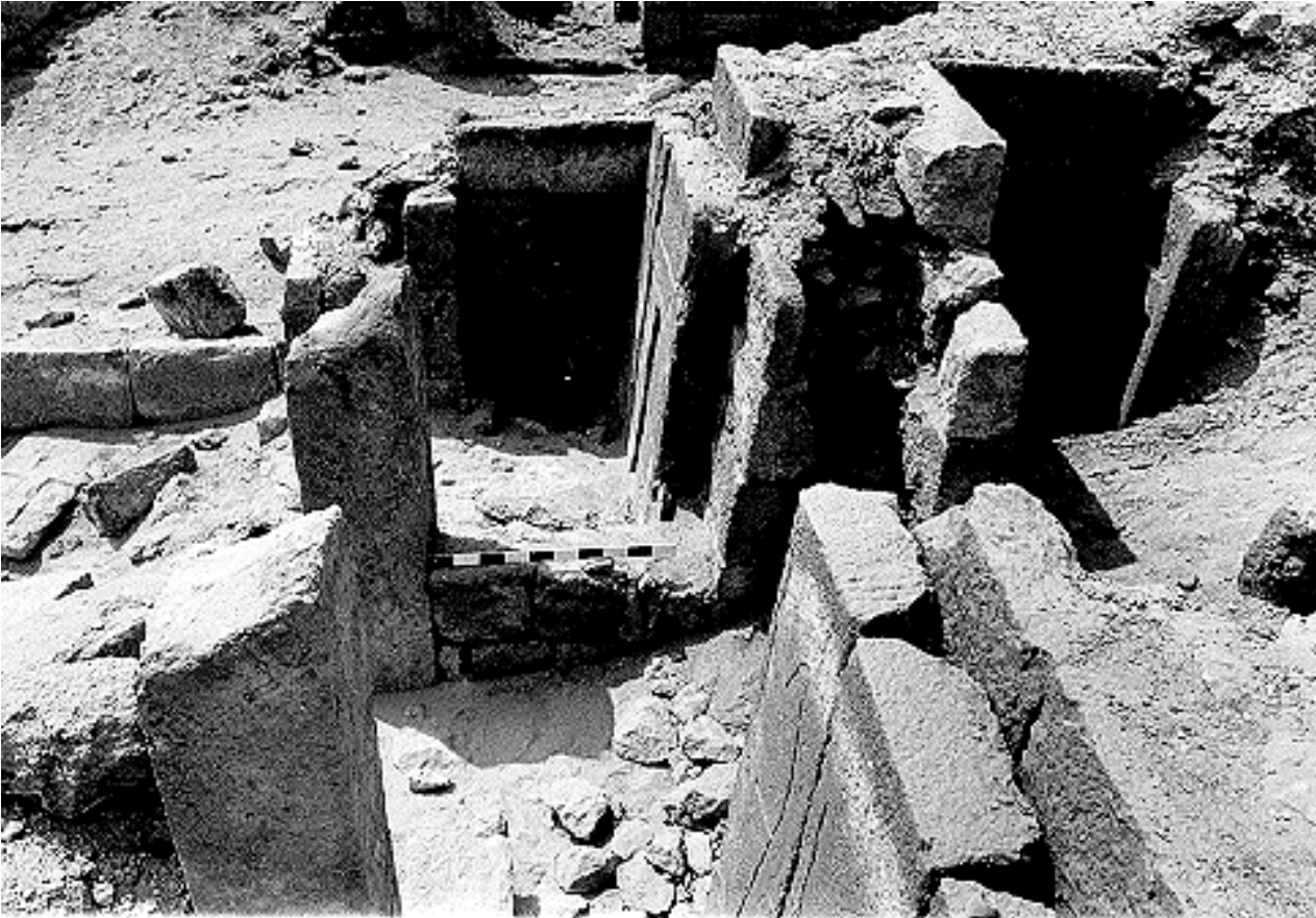
27a. 2088: portico from the north, showing the ashlar block facing added to make its back face somewhat more vertical. (The false door, however, retained the angle of the underlying facade.) The wall under the photo scale is part of the intrusive mastaba 2088a. The L-shaped chapel and its southern false door can be seen to the right (rg 14-24, 1989)
