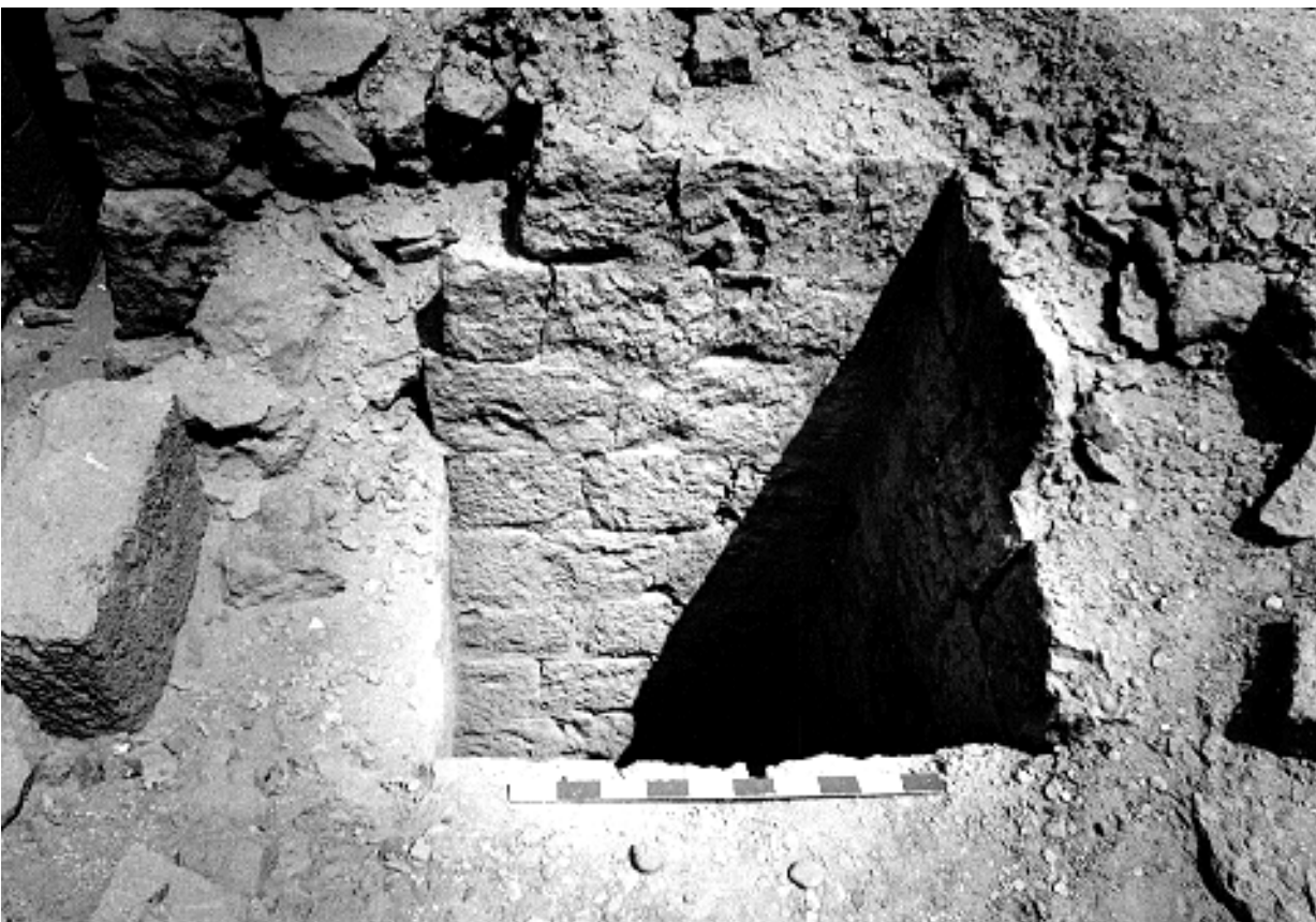
60b. 2091 a: top of shaft. Footholds have been cut down the center of the north face. (The other three faces have similar footholds) (rg 23-13, 1989)
